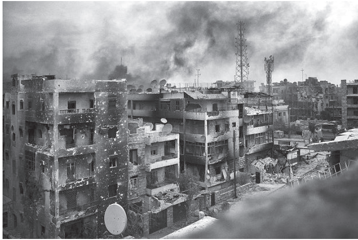
Bombed-out buildings in Aleppo, October 3, 2012, show the devastation perpetrated on civilians. The Assad regime's brutal response to the revolt has only widened the circle of rebellion. Many who have joined the fighting are motivated by the desire to take revenge for the spilled blood of their relatives or the destruction of their homes and communities.
